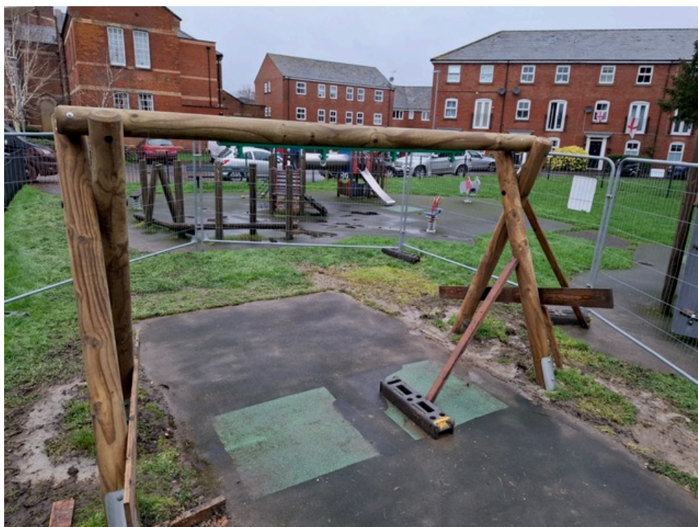
Figure 5: Scheduled replacement works at Hillier Road, showing investment in new equipment.
